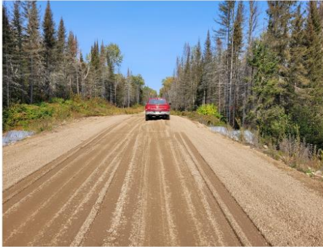
2. South Approach (looking north)
