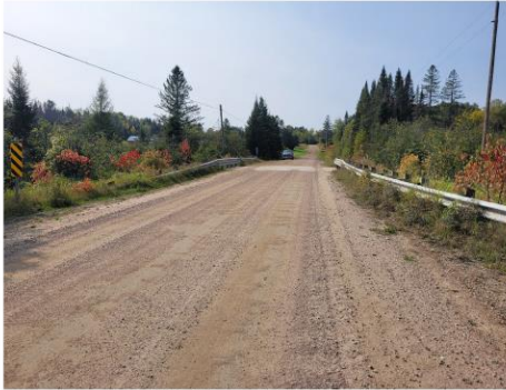
1. East Approach (looking west)
