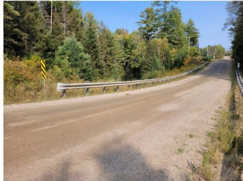
4. North Barrier (looking east)
