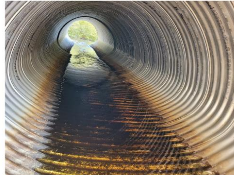
6. Inside South Barrel (looking east)
